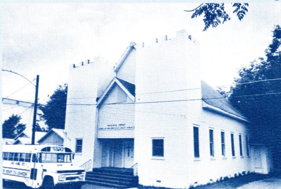
960 KANE (Ca. 1935)—The oldest church structure of the eight in the district. 3x6-bay concrete block structure with central gable and square tower which terminate crenelated battlements. Recessed entrance. Exposed rafter-tails.
