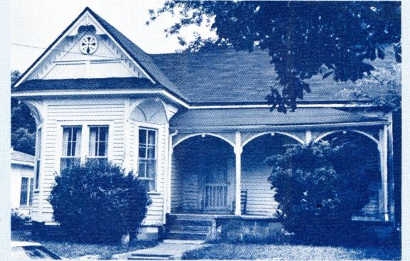
154 E. DAVIS (Ca. 1890)—Queen Anne style. 1-story, L-plan cottage with elaborate gable treatment; diagonal beaded board; cut-out vergeboards, round ornament with pinwheel design. Porch posts connected by latticed arches.
