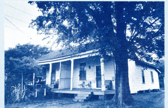
154 W. MONUMENT STREET (Ca. 1860)—A creole cottage style with undercut gallery and paneled Greek Revival posts 6-over-6 sash.
