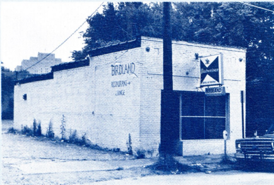
524 N. FARISH (Ca. 1928)—Birdland Lounge—commercial building with corbelled cornice. Soldier brick belt course above storefront and decorated frieze. Floral tie rod caps.
