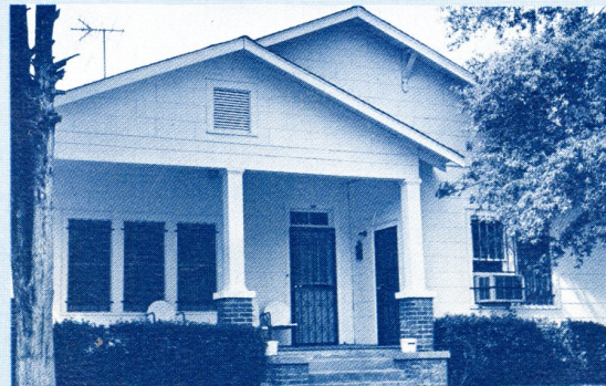
226 E. OAKLEY (Ca. 1930)—bungalow style; 1-story 3x3 bay front-gabled house with exposed rafter-tails and bracketed front eaves. Two gabled porch on square posts. Triple and double windows.
