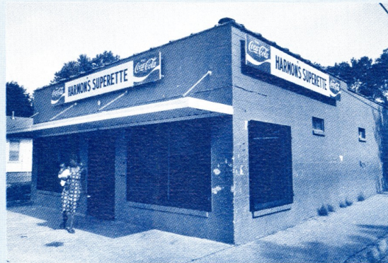
158 E. MONUMENT (Ca. 1935)—concrete block store with tile covering. Central entrance with double leaf door.
