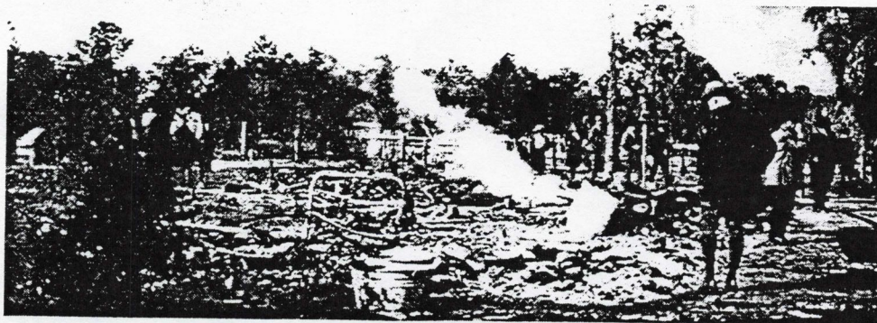
Aftermath of 1923 fire.
